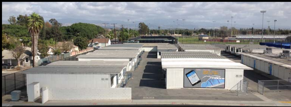
BEFORE PORTABLE DEMOLITION
